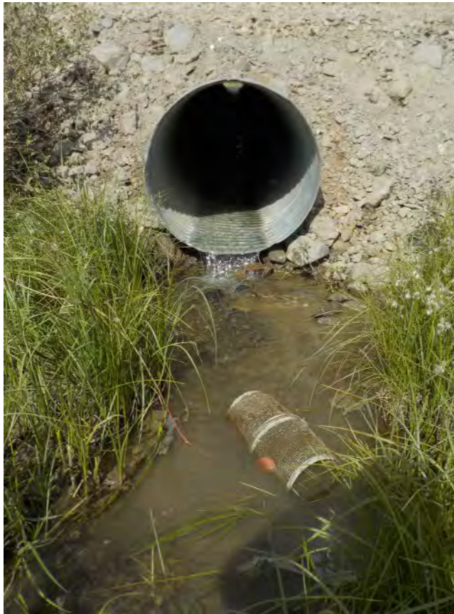
P_F86AY002_007_DS CULVERT 7/16/2015 AL145.3 PHOTO OF PERCHED CULVERT DS OF FT & MINNOW TRAP 3
