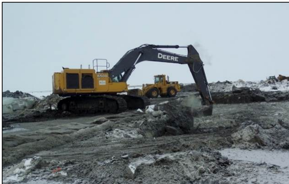
Figure 4-9. Ice Removal at Site #1
