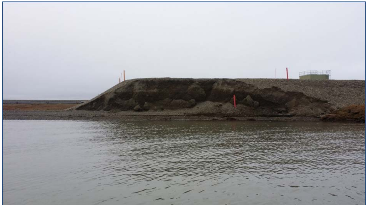
Figure 4-7: Photograph of WEST Showing Erosion of AGI Pad
