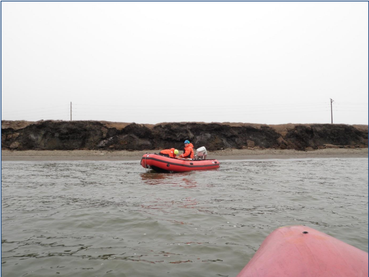
Figure 4-6. Photograph of Site 1 – SBAY Showing Shoreline Erosion
