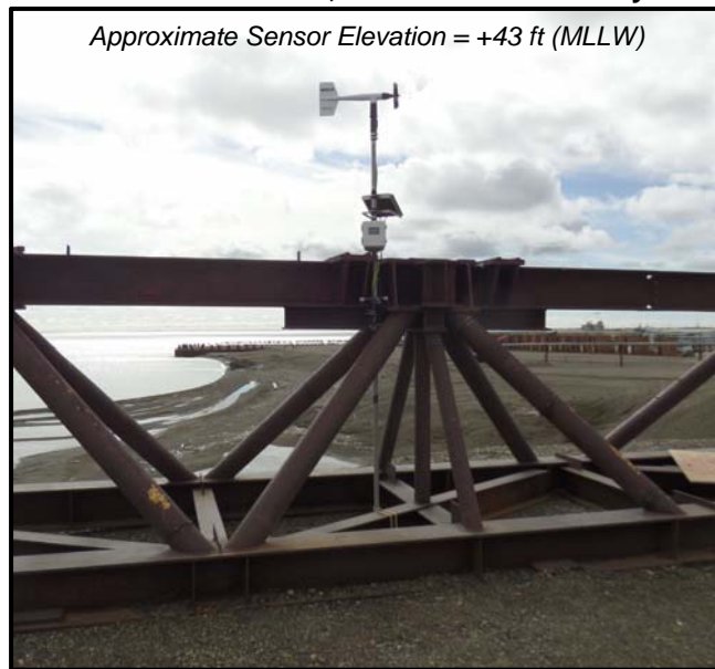
Figure 3-1. Anemometer Installation, West Dock Causeway 52-ft Breach (2016)
