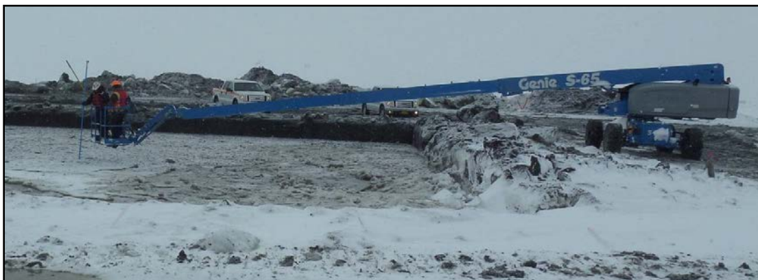
Figure 4-14. Use of Man-lift to Survey Test Trench
