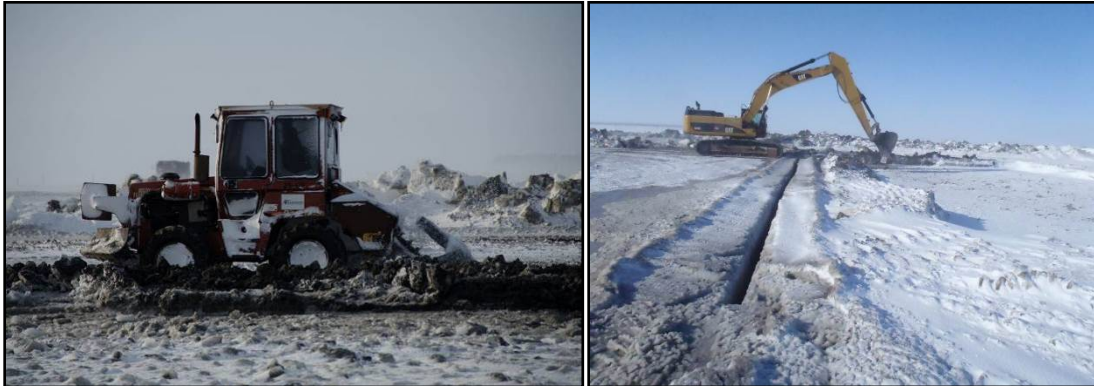
Figure 4-8. Trencher Slotting Ice (left) and Ice Slot (right)
