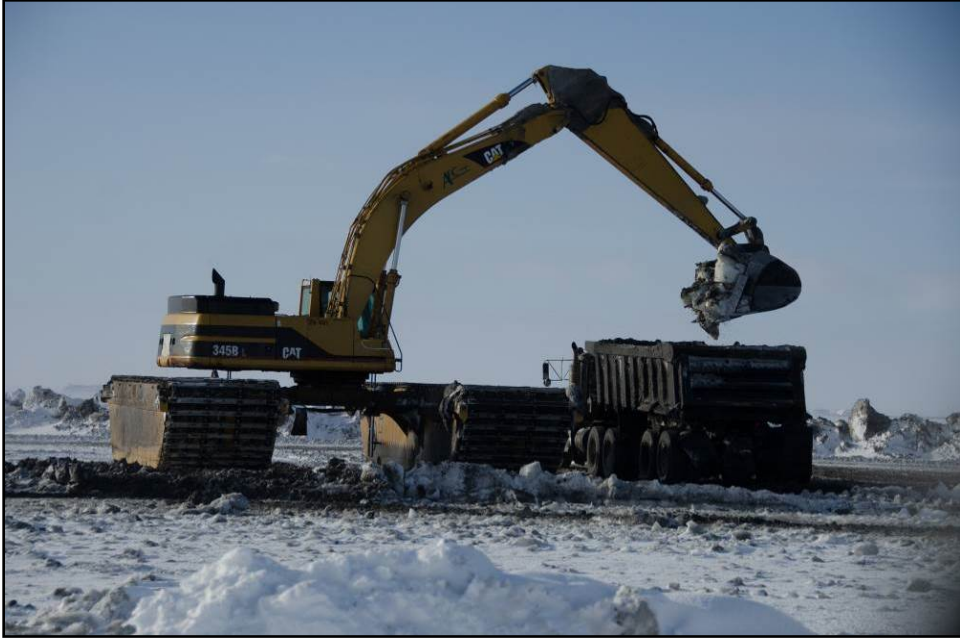
Figure 4-10. Ice Removal and Hauling at Site #2.5
