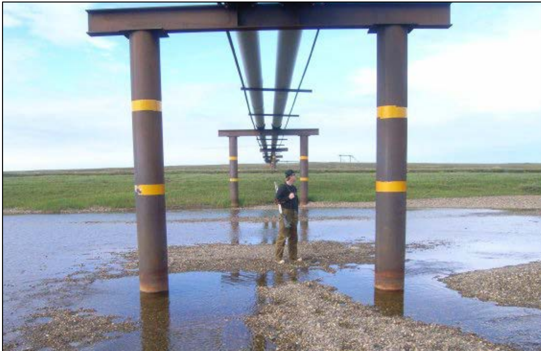
Figure 14: Support Piers at the Miluveach River Crossing
