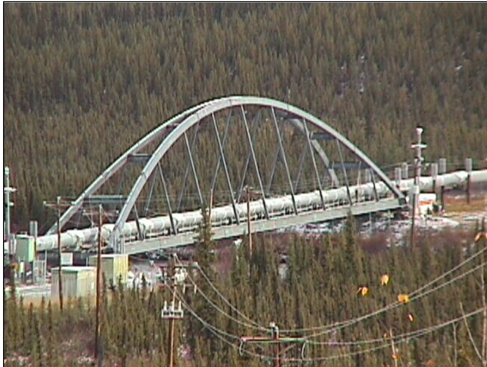
Figure 6: TAPS Crossing of the Gulkana River
