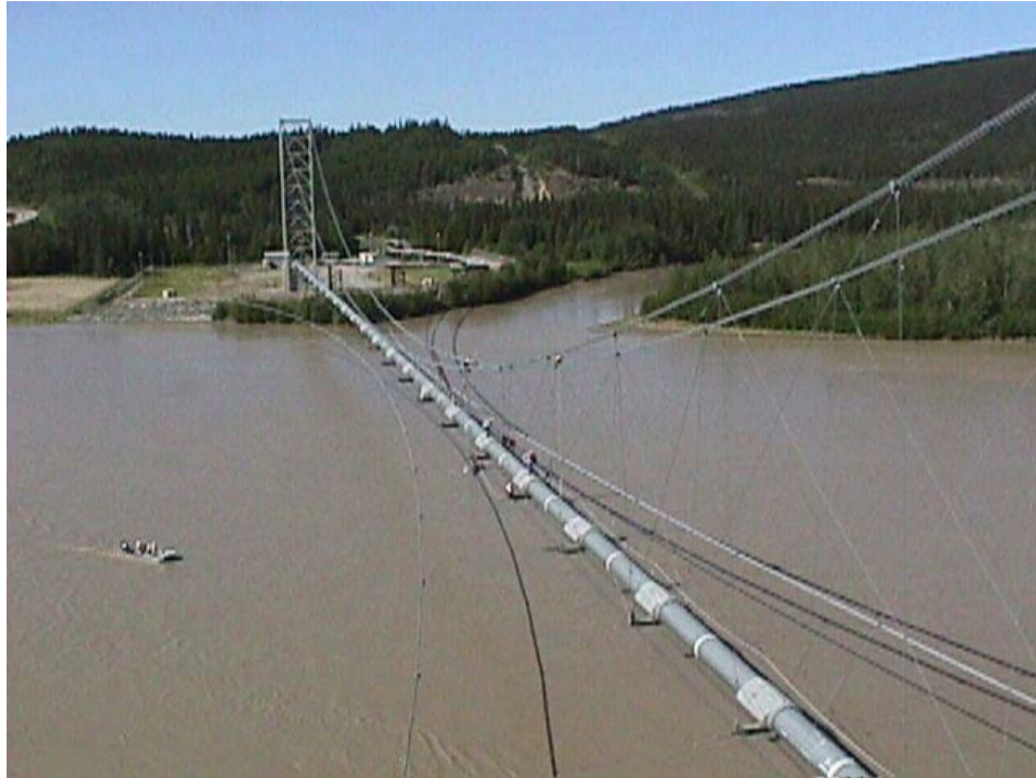
Figure 12: TAPS Pipeline Suspension Bridge over the Tanana River
