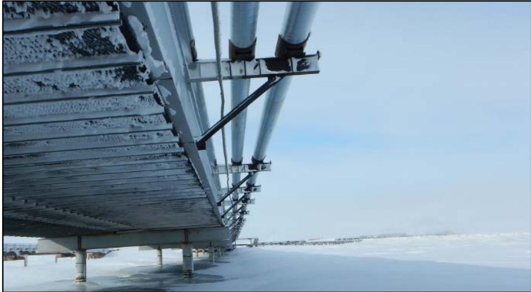
Figure 20: DS 16 and DS 17 Pipeline Beam Extensions
