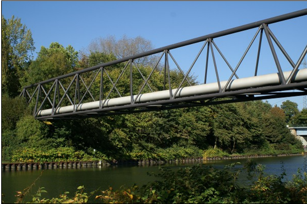
Figure 10: Pipeline Truss Bridge
